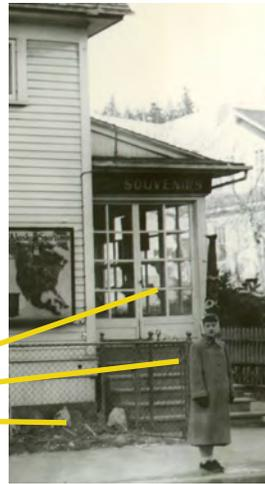
In considering the existing and required level of accessibility, it is clear that there is not an accessible entry available (the first floor level is approximately 42” above grade and sidewalk level). A ramp will be required that will need to be approximately 42’ in length to meet ADA slope requirements. This will be a difficult accessibility requirement to meet given existing configurations of entry doors, interior corridors, public restrooms, and other barriers.
