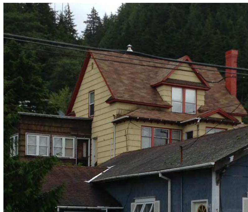
The addition on the west, which also wraps around the back of the house, employs a different roof pitch, fenestration treatment and paint color than the rest of the house.
