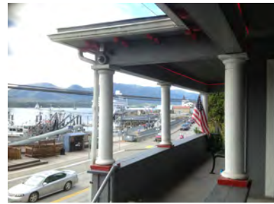
Raking cornice and doric columns
