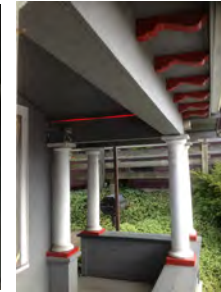
Raking cornice and doric columns
