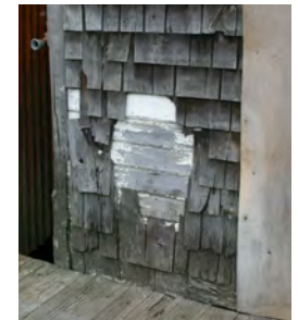
Original siding under cedar shingles
