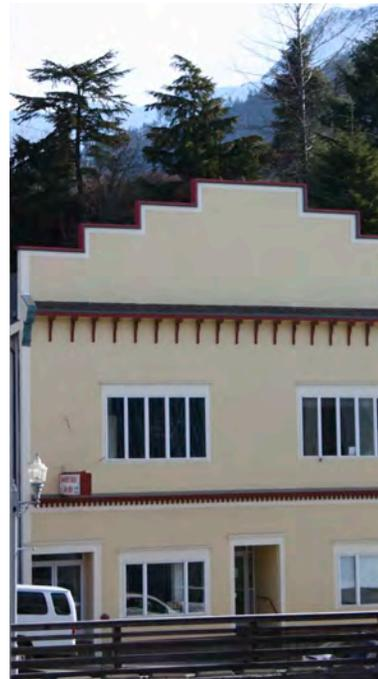
*By 2011, many historic architectural features were still evident. The original windows were replaced, some were removed, and sidewalls were clad with metal siding; but the character defining features (stepped parapet and cornice) remain.*
