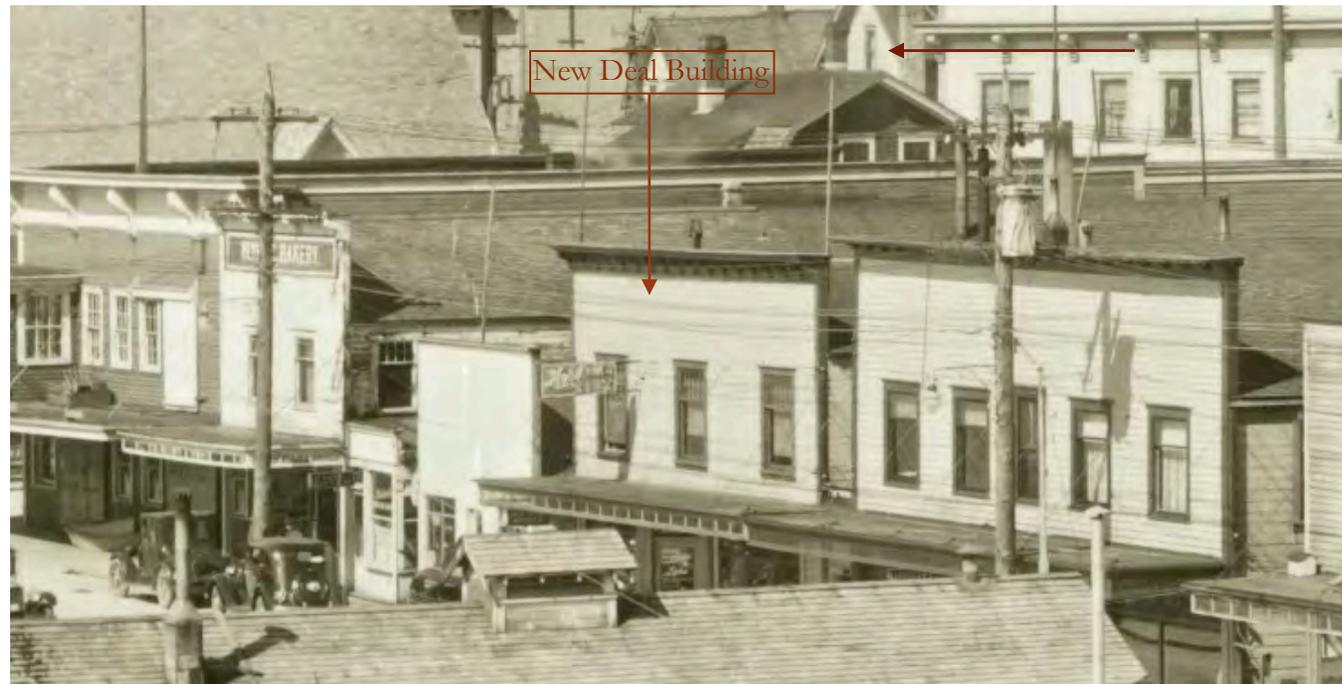
*This early-1930s partial view of the New Deal building shows a bracketed cornice, a marquee with divided lites and similar window placement as today. Not long after the building was constructed, the cornice was removed and a triangulated parapet was installed that remains on the building today.*
