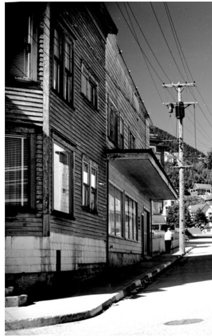
*These photos (left, 1952 and right, 1954) show the period window openings and facade treatment that survived into the 1960s. The portion with the marquee is an addition to the original building that carried the facade all the way to the street.*
