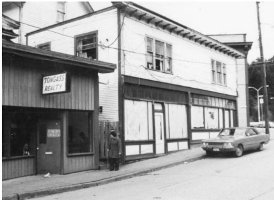
*This 1977 photo of 435-439 Dock Street shows the original bracketed cornice along the full length of the building, the two sets of three double-hung windows on the street front, and the storefront facade with its transom windows. The bracketed cornice remains today.*
