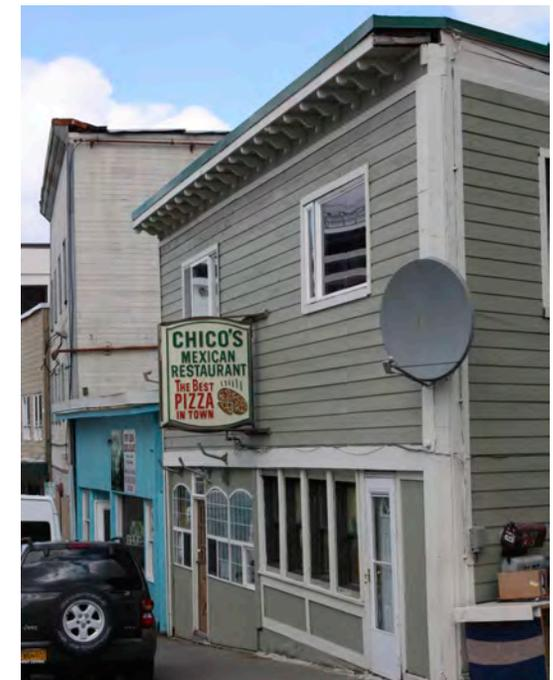
*While recently sheathed in non-period wood siding, Chico's retains its original massing, cornice and corner boards.*
