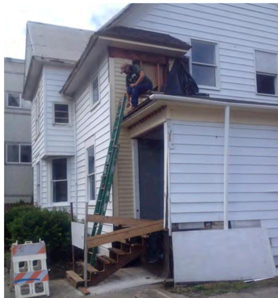
*As shown in this August, 2013 photo, the east and south (Mission Street) elevations have a vinyl siding cover added in the 1970s. As part of the historic building assessment, a portion of the vinyl siding was removed to expose the original cedar siding and determine its condition for restoration. The original siding is still in excellent condition and needs only minor repairs.*
