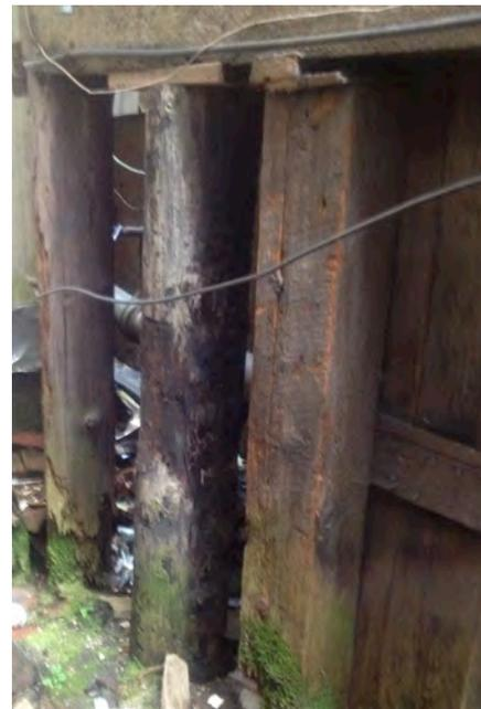
*Piling conditions at the west elevation. In this case (and it is typical), a new creosote pile was placed between two adjacent deteriorated piles to carry the building load. There is no attachment between the piles and the cap.*
