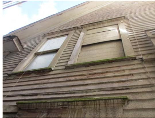
*On the west facade, the original cedar siding was not clad in vinyl but received a treatment of sprayed-on plastic material. All of the original fenestration detailing remains. This elevation is protected from the elements and shows little deterioration.*
