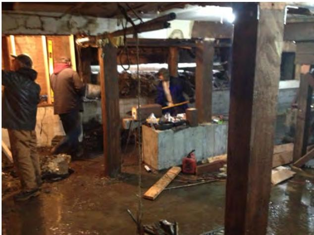
Historic Ketchikan recently completed a temporary stabilization project in the partial basement area. A shear wall was installed on the existing concrete stub walls and 8 new piling were installed with steel angles connecting the piling to the piling caps.
