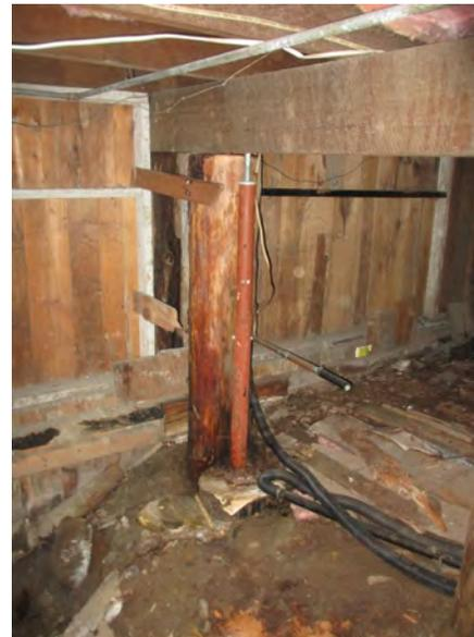
*The log posts supporting much of the building are significantly deteriorated. In many cases, they have been augmented by screw jacks, as shown here. The 8x10 heavy timber piling caps are in generally excellent condition.*
