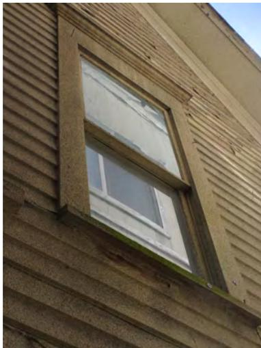
*On the west facade, protected from the weather and remodelers, all historic windows remain in the various configurations occurring on the other facades, and all detailing is intact. These windows can serve as the model for replacing any of the period details on the south and east facade windows.*
